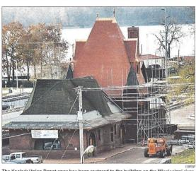
The Keokuk Union Depot apex has been restored to the building on the Mississippi riverfront. Tiles made by the original manufacturer and finials are installed. The next roof work will include the upriver and downriver wings of the building.
