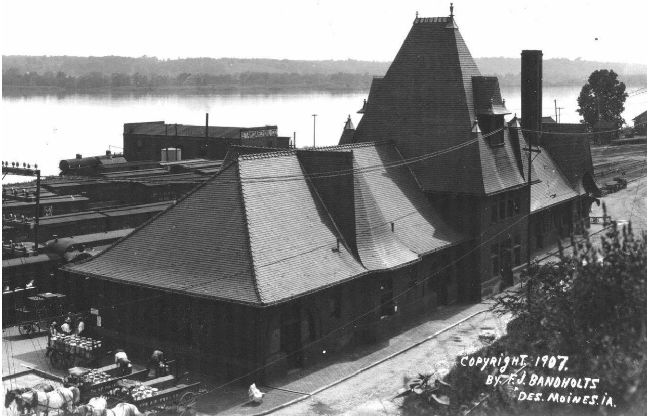
Fig 14. The Depot's original roofline and all of its decorative accessories.
