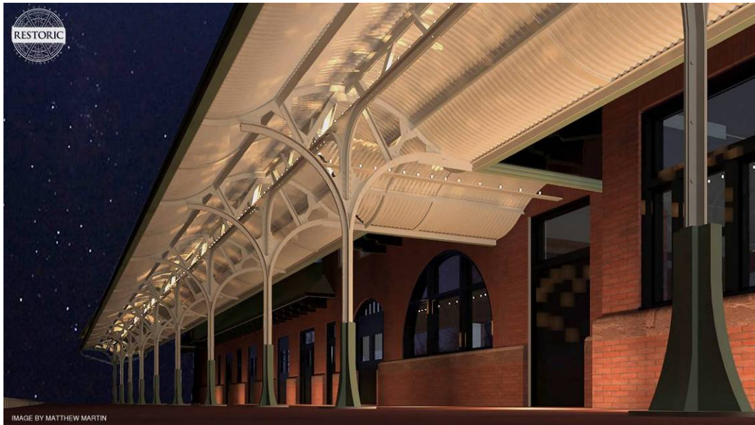
Fig 28. A 2014 rendering of the trackside canopy with restored “marquee” style strip lighting.
