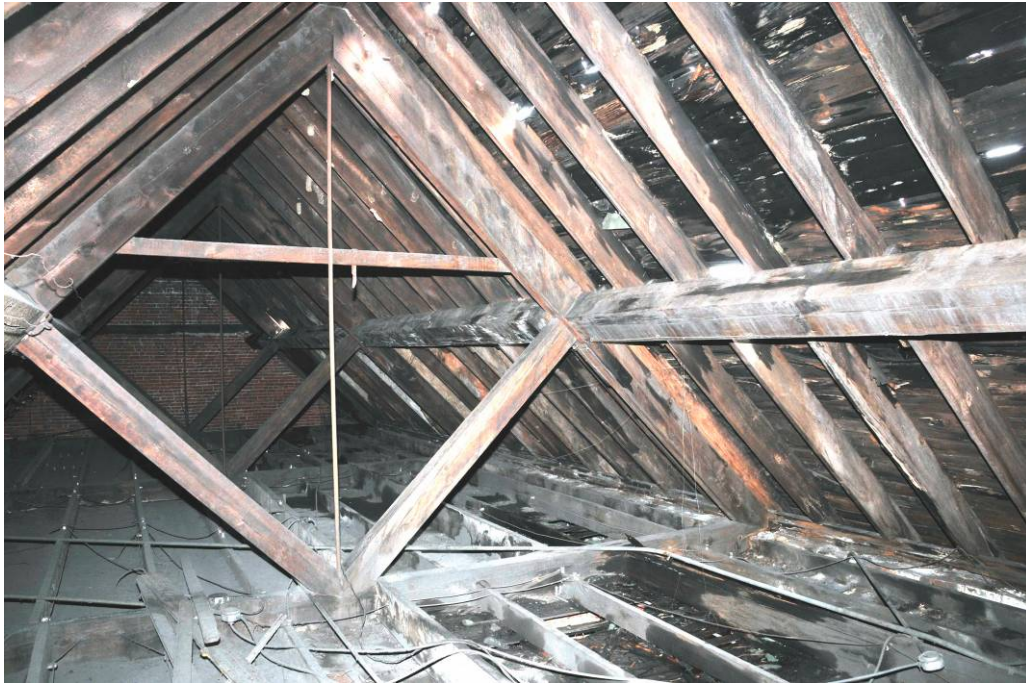
Fig 20. View upriver of riverside slope roof framing over the freight rooms.
