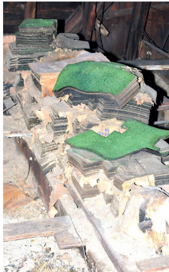
Fig 17. Stockpile of asphalt shingles.
